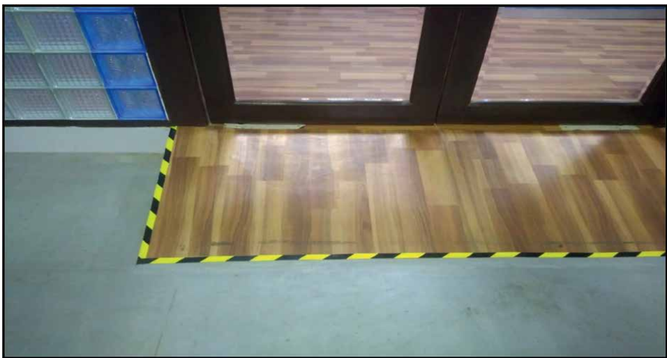
Figure 7. Safety sign indicator.
