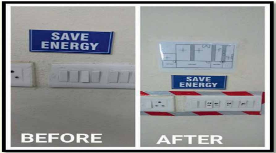
Figure 5. 2S – Labeled switches in the campus.
