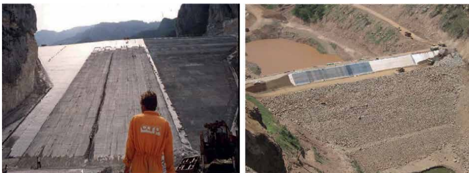
Figure 11. At left Bovilla dam, at right Gibe III 50 m high cofferdam.
