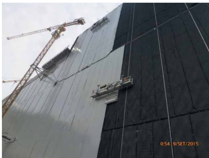
Figure 3. Susu RCC dam. From right to left, the vertical U profiles fastened to the dam, the black drainage geonet placed between them on the upstream face, the waterproofing liner being placed on the geonet, some Omega profiles providing temporary anchorage against wind uplift, and at the extreme left the Omega profiles permanently fastened.
