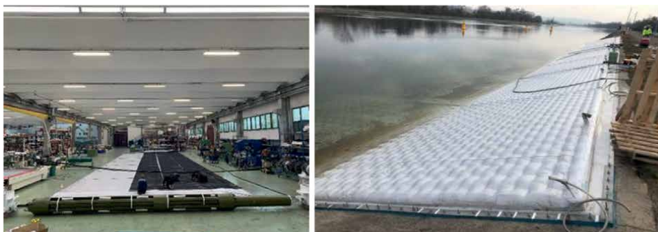
Figure 15. The SIBELONMAT® panels under fabrication (at left) and injected and sealed at Kembs dike, part of the Grand Canal d'Alsace navigation canal in France.
