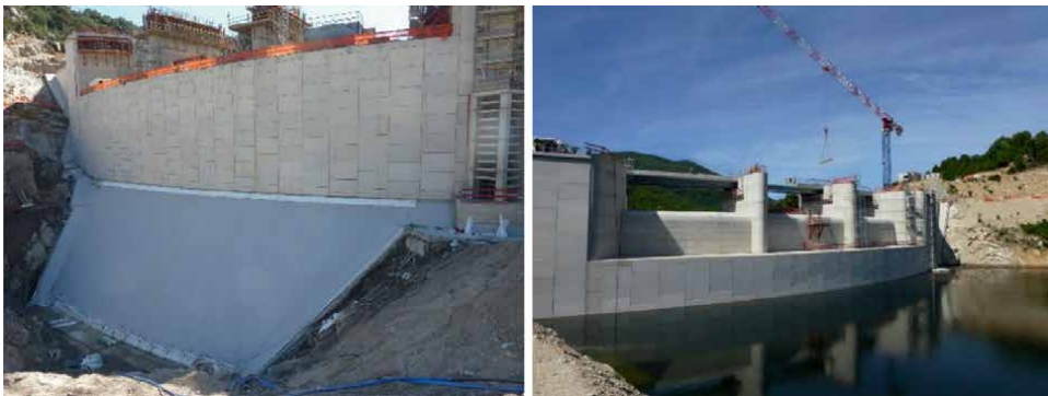
Figure 6. Rizzanese dam. Placing the geocomposite at the inclined section before covering it with anti-puncture geotextile and backfill (left), and the impounded dam.
