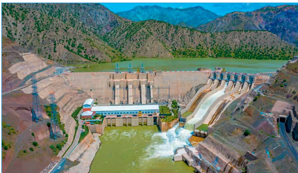
Figure 4. A general view from the Upper Kalekoy Dam.
