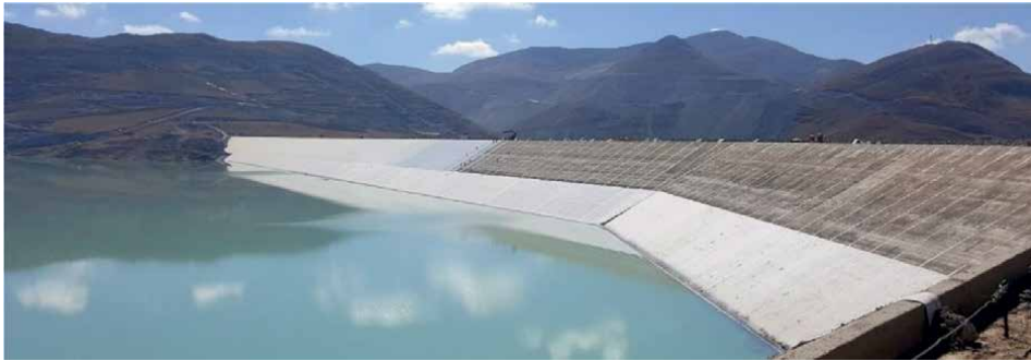
Figure 8. Staged installation on curbs at Las Bambas dam, now reaching 173 m.
