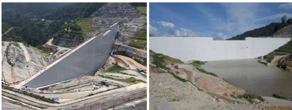
Figure 4. View of the upstream face of Susu RCC dam at completion of the geomembrane system at spillway (left), and at start of impoundment (right).
