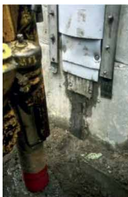
Figure 13. Detail and view of external waterstops installed at monolith joints of Platanovryssi 95 m high RCC dam in Greece.
