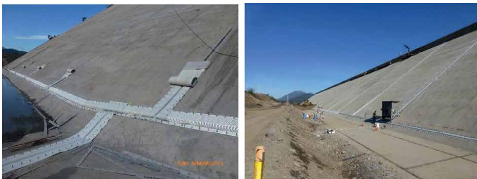
Figure 14. High-tech support textile and waterproofing geocomposite at Angostura 32 m high 1.6 km long concrete face gravel dam, Chile. External waterstop on peripheral and vertical joints designed to resist joint openings up to 300 mm.
