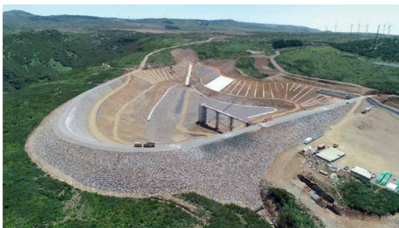
Figure 10. Installation of waterproofing liner over anchor trenches at Pico da Urze dam.
