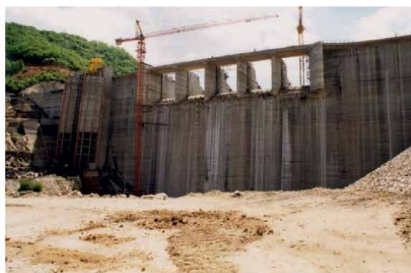
Figure 13. Detail and view of external waterstops installed at monolith joints of Platanovryssi 95 m high RCC dam in Greece.
