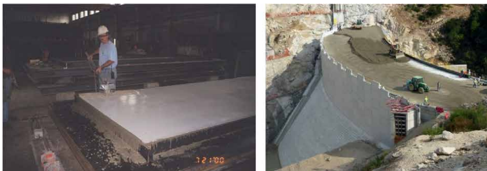
Figure 5. Vibrating the concrete to attach the geocomposite to the precast panel (left), and Rizzanese RCC dam seen from the upstream: the bottom inclined section has not yet been lined, placement of RCC against the panels with embedded geocomposite + protection geotextile at the vertical section is ongoing (right).
