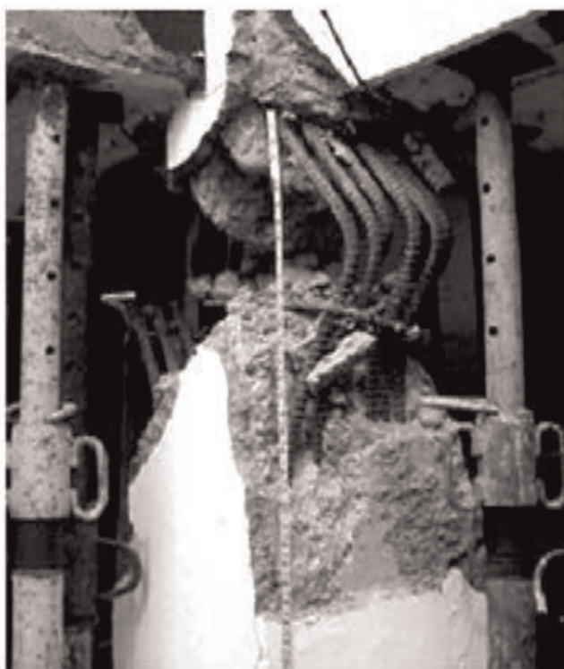
Figure 2. The severe failure in the column due to large distances of transverse reinforcements [3].
