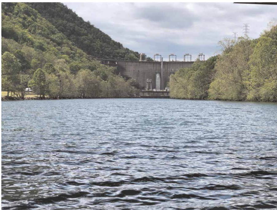
Figure 2. Smith Mountain Lake reservoir dam shown from the pump storage reservoir Leesville Lake located in Central Virginia. This pump storage operation pumps water from Leesville Lake during off peak to generate power during peak from Smith Mountain Lake.
