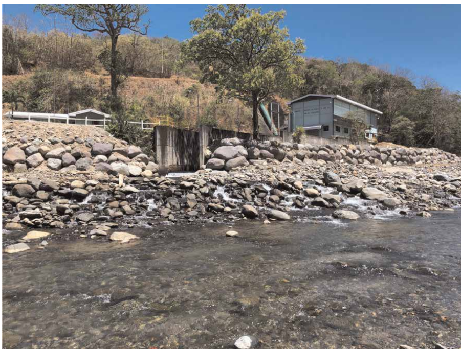
Figure 1. Hydropower plant located along Rio Aranjuez in Costa Rica. This power plant diverts water from the river above to drive turbines for electricity production. Power generation is completely dependent on adequate flow from the river.
