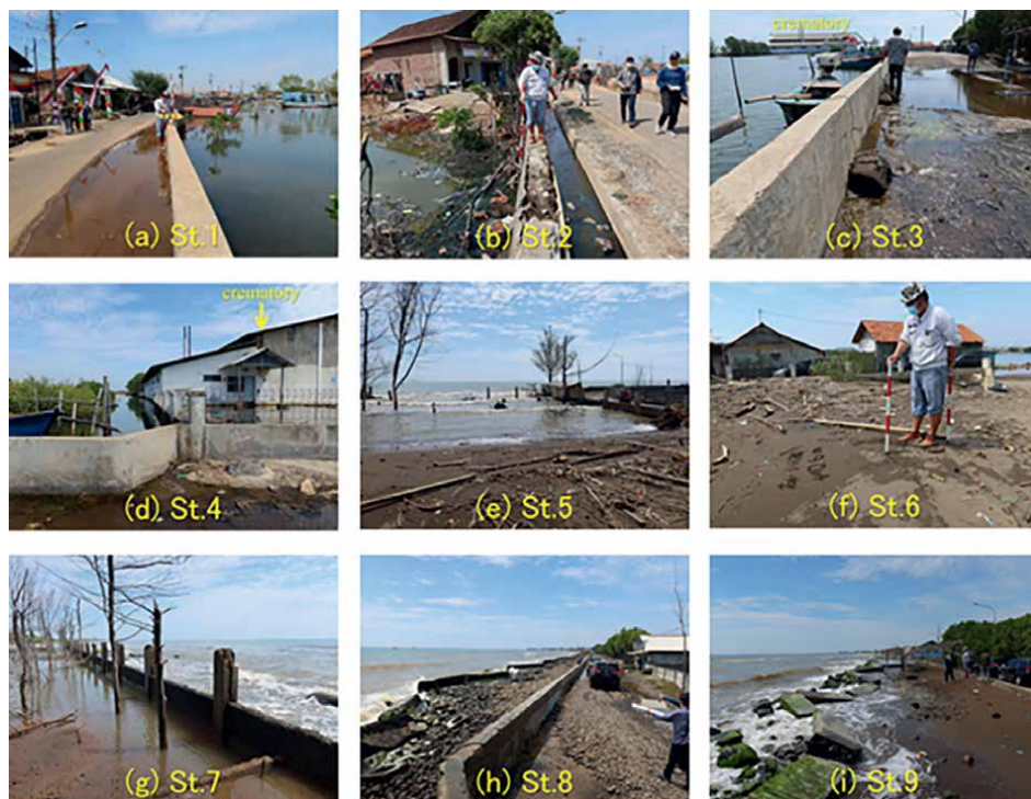
Figure 4. Photographs showing ground subsidence taken at Sts.1–9 in Pekalongan.
