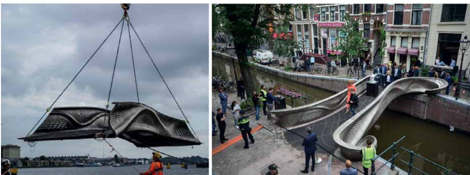
Figure 4. 3D-printed pedestrian bridge in Amsterdam, Netherlands, built in 2021.
