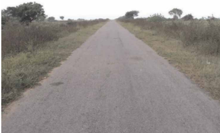
Figure 1. View of a typical low-volume road in India.
