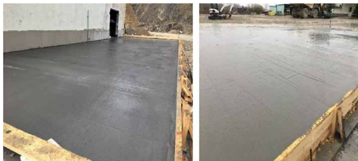
Figure 5. View of the CSS and ACBFS concrete pavement.
