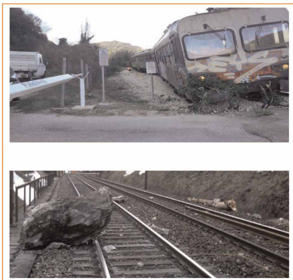
Figure 5. Accidental obstacles on a railway site.
