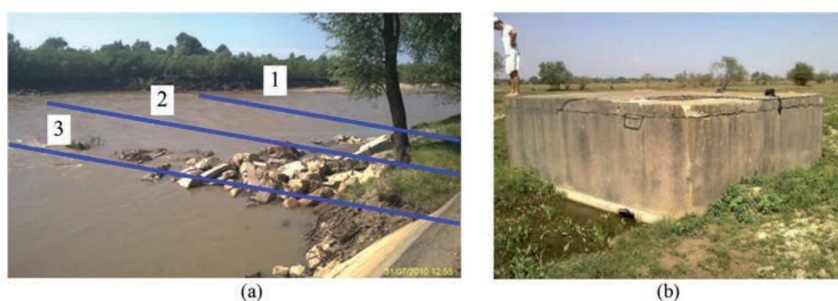
Figure 6. The characteristics of the undercrossing construction on the Moldova River: a – scheme for the location of the pipelines on the left arm of the river, 1 – Ad1, 2 – Ad2a, 3 – Ad2b; b – the CV2 chamber with the hydraulic installation on Ad2b [19].
