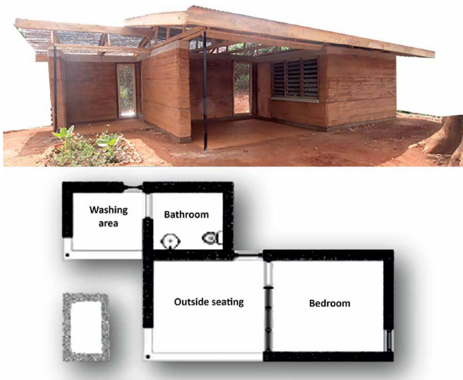
Figure 3. The Nkabom House: a model for sustainable earth construction and recycling in Ghana.
