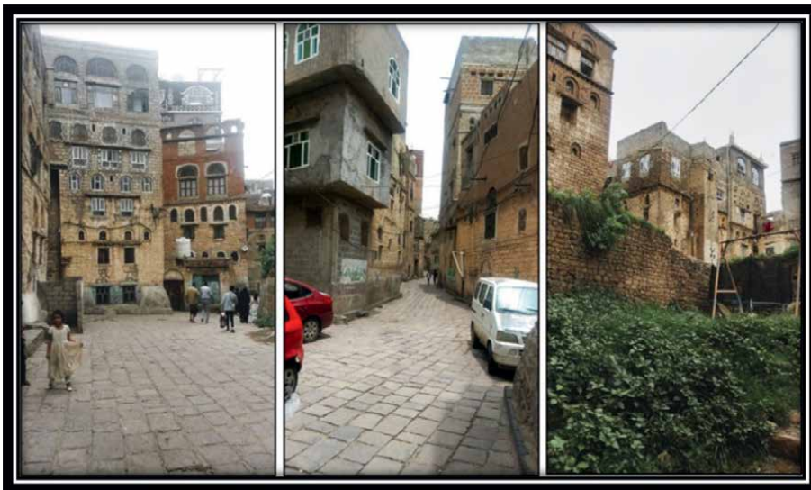
Figure 20. Demolishing and replacing Ibb City's historically houses.
