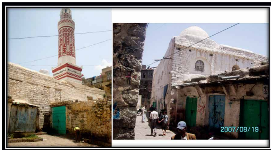
Figure 2. Show Al-Jalalia higher school structure (closed school).
