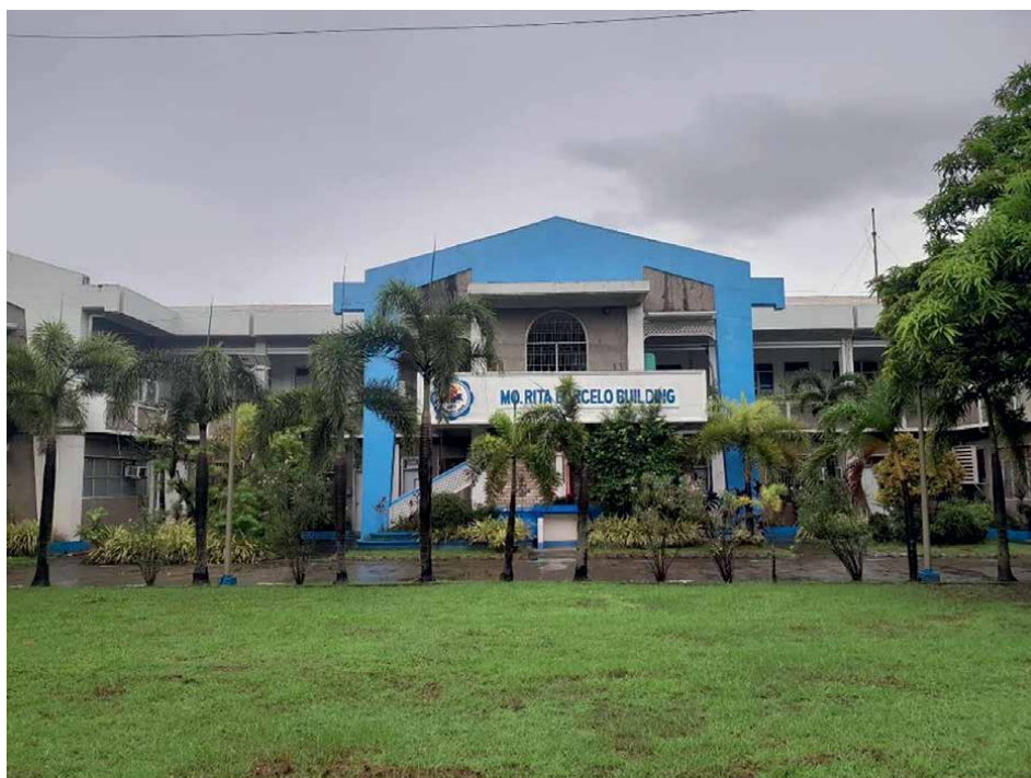
Figure 6. La Consolacion University Philippines-Catmon campus Mo. Rita and Mo. Consuelo buildings.
