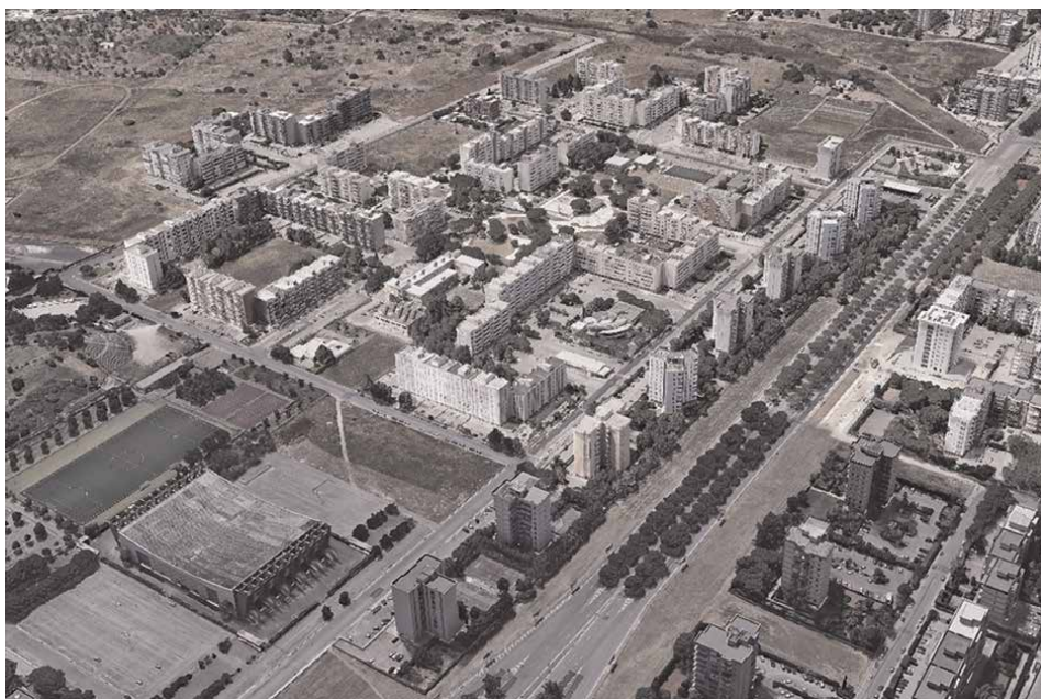
Figure 2. Compound of Caldarola 45, aerial photo.
