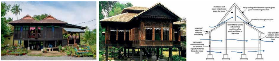
Figure 1. Elevated floors in traditional Malay house.
