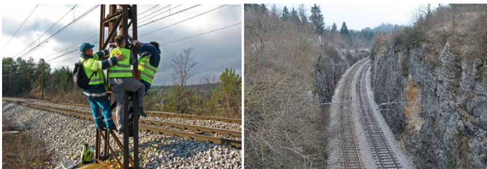
Figure 1. Installation of acoustic deterrents on electric poles (left) and part of railway tracks with higher risks of collision with train (right) (foto: M. Zaluberšek, 2016 and K. Kotnik, 2020).
