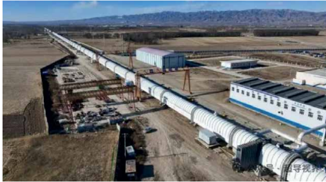
Figure 21. The first phase of the China high-speed flying car system test line by the CASIC [37].
