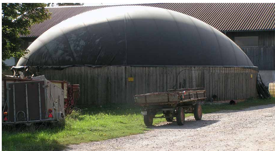
Figure 10. Single-layer membrane cover made of EPDM [© Rosemarie Wagner].
