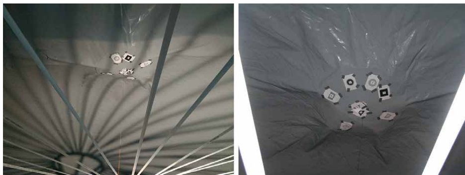
Figure 19. Geometry of the gas membrane during gas production caused by the weight of the pol cap [© Rosemarie Wagner].
