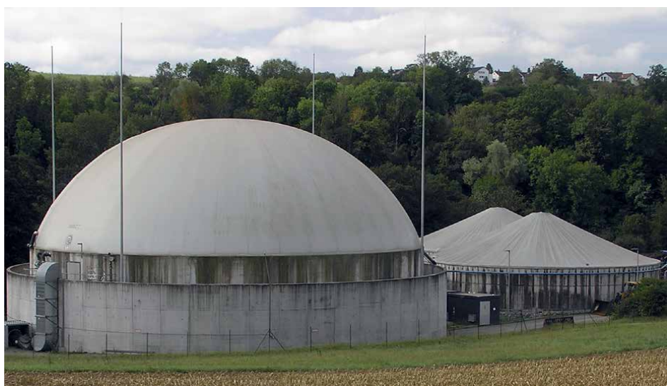
Figure 1. Typical membrane covers at biogas plants [© Rosemarie Wagner].
