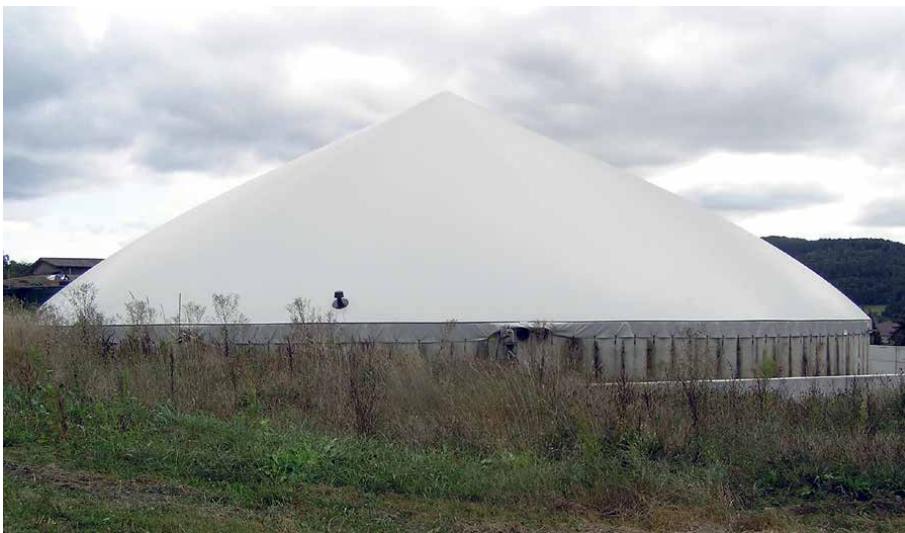
Figure 3. Cone-shaped membrane as internal pressure-supported structure [© Rosemarie Wagner].
