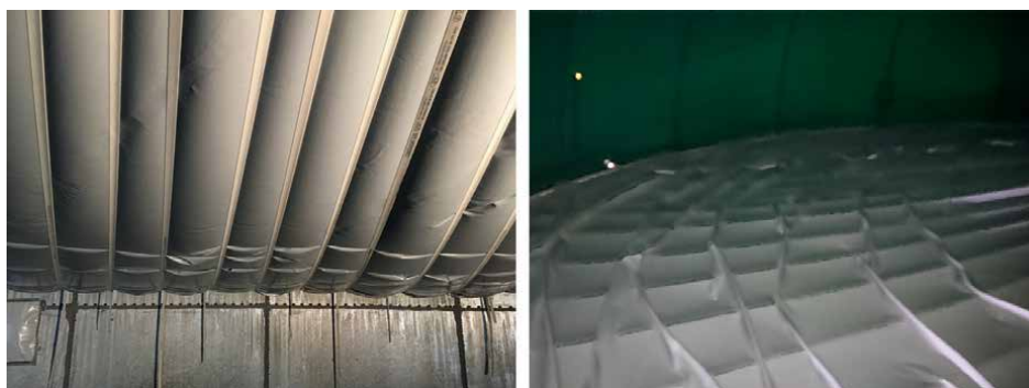
Figure 23. Gas membrane, loaded with pressure in the air-supported volume and negative pressure in the gas volume, from below (left) [© Rosemarie Wagner] and from above (right) [© Kai Heinlein] the gas membrane.
