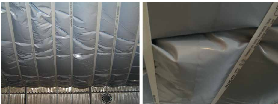
Figure 18. Depositing the gas membrane onto a belt system [© Rosemarie Wagner].
