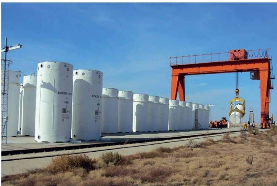
Figure 4. Photograph of a dry cask storage site in the U.S. Source: U.S. NRC [10].
