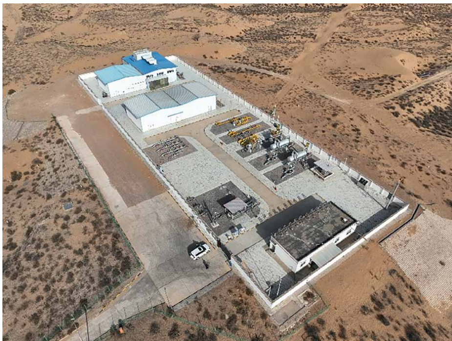
Figure 1. Sulige gas field gathering station.
