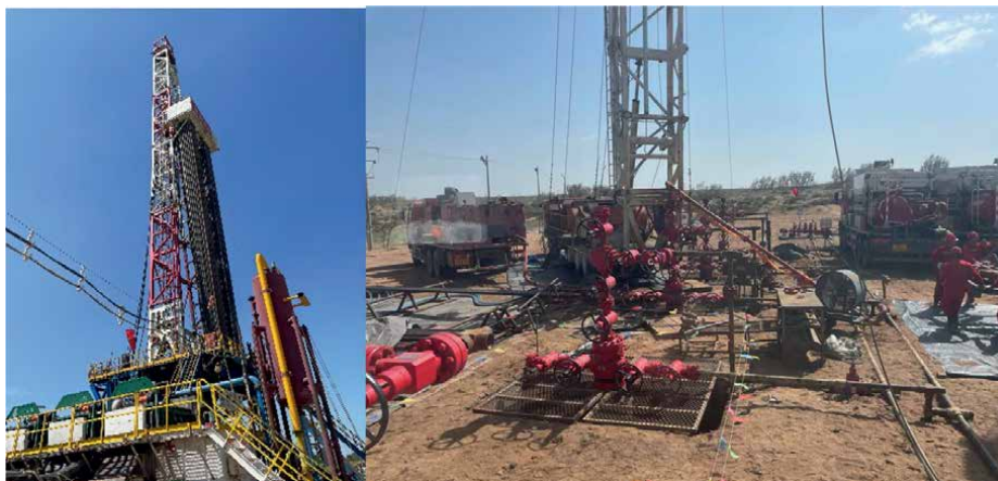
Figure 2. Drilling and hydraulic fracturing sites at sulige gas field.
