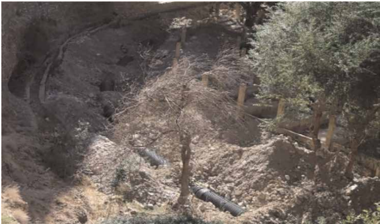
Figure 5. The buried sewerage HDPE pipeline is raising the sewerage outfalls of the Barada River in Syria.
