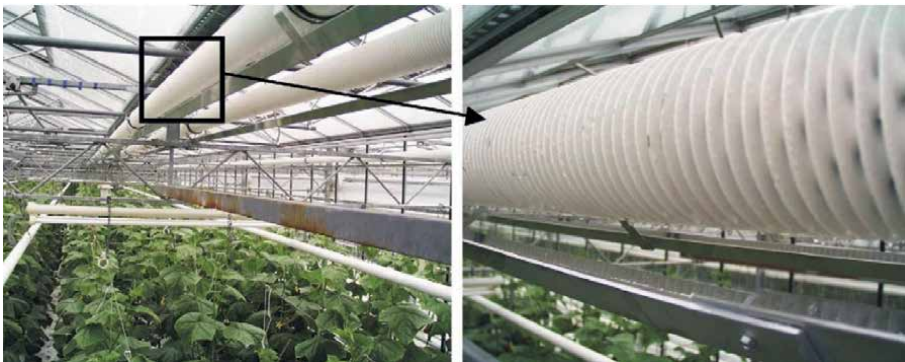
Figure 5. Photograph of the greenhouse where finned tubes are placed under the gutter and an enlargement of a finned tube with condensation on the surface Campen and Bot [64].
