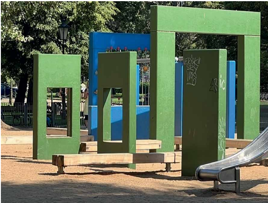
Figure 9. Constructed wall panels for a built form playground. Panels for spatial separation in the playground. Source: Watts.
