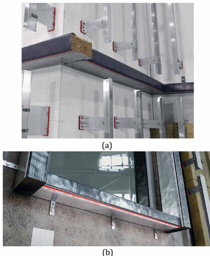
Figure 7. (a) Photograph showing the joints of a typical cavity barrier system and (b) supports used to fix cavity barriers to walls [20].
