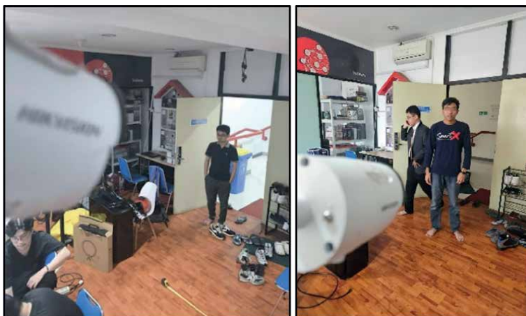
Figure 2. Example of installing CCTV indoors.
