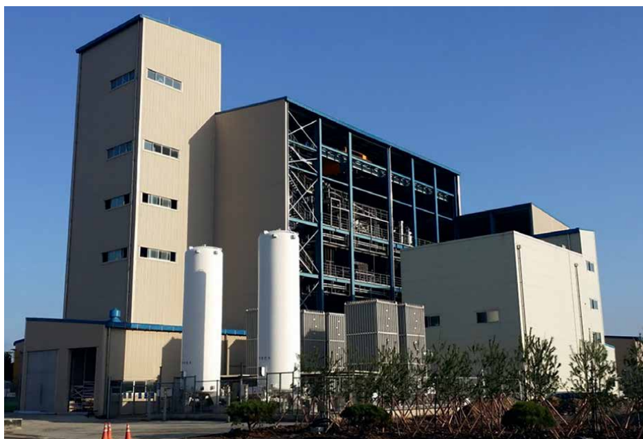
Figure 15. Overview of demonstration scale plant for hydrogen production using pet-coke.
