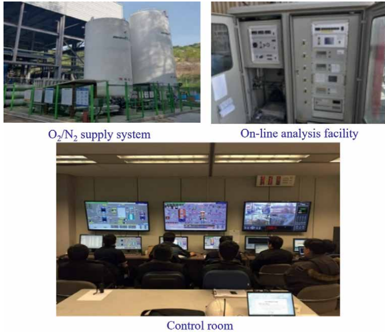
Figure A2. Utilities supply, syngas analysis systems, and control room view of pilot-scale (2 ton/day) plant.
