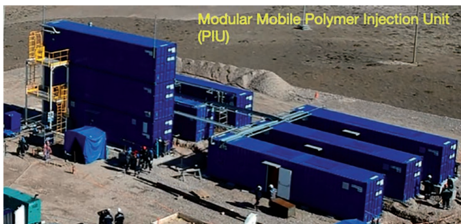
Figure 6. Modular mobile Polymer Injection Unit (PIU) used for Enhanced Oil Recovery (EOR) operations in remote locations. The PIU is composed of stackable, interlinked container modules, enabling rapid deployment, flexible relocation, and minimized site preparation. This setup supports polymer preparation, dosing, and injection without the need for permanent infrastructure [1, 29].
