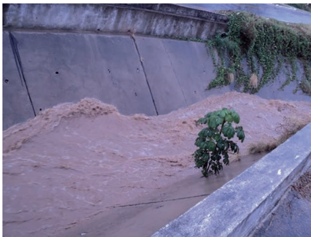
Figure 2. Supercritical flow in the Granjeiro stream channel in the initial urban section upstream of the entrance to the first storm drain (The Author, October 19, 2011).
