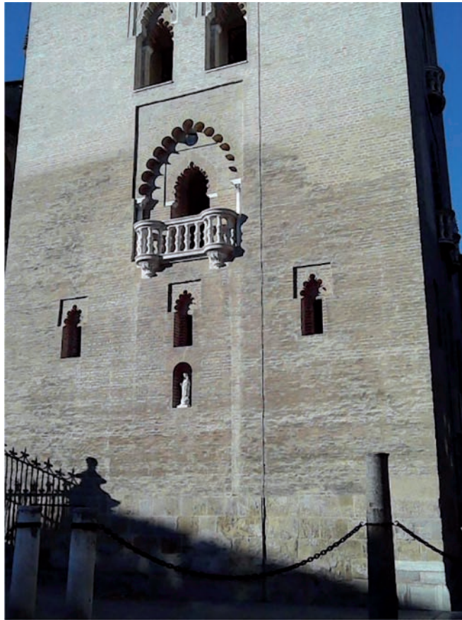
Figure 15. Photographic image of the lower eastern facade of La Giralda in Seville Cathedral, revealing moisture issues (photo by the author).
