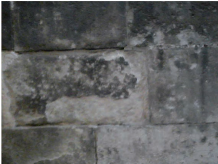
Figure 19. Black crusts on the sandstone ashlars of the facade of the Cathedral of Barcelona (photo by the author).
