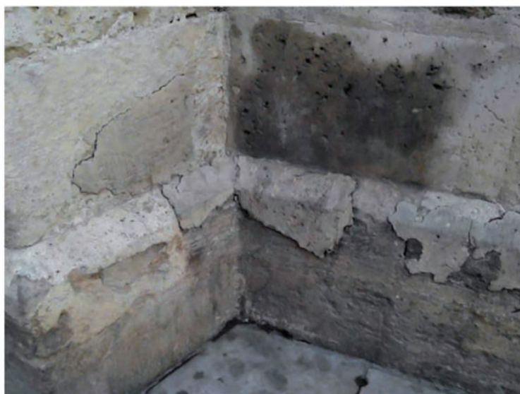
Figure 17. Detail of the southeast facade base of the Torre del Miguelete in Valencia Cathedral, showing diverse materials and varying deterioration states (photo by the author).
