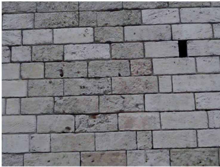
Figure 11. Detail of the south façade wall of the Cathedral of Palma de Mallorca, where different ashlars from the Marés can be seen (photo by the author).
