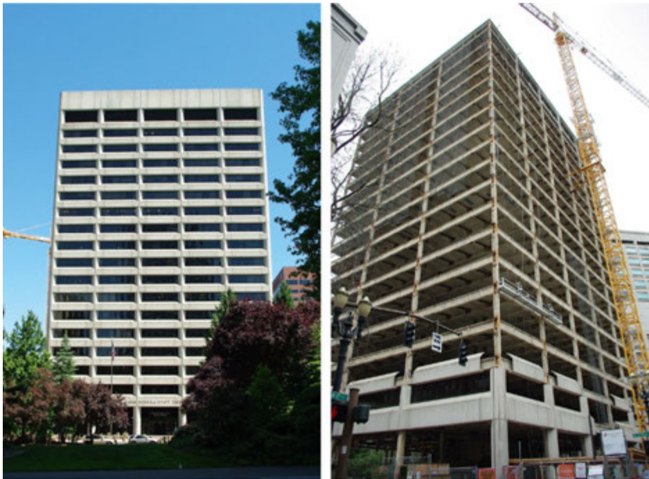
Figure 1. The Edith Green - Wendell Wyatt Federal Building in 2008 before renovation (Left) and during facade removal in 2011 (Right). Images: CC-BY-SA M.O. Stevens.
