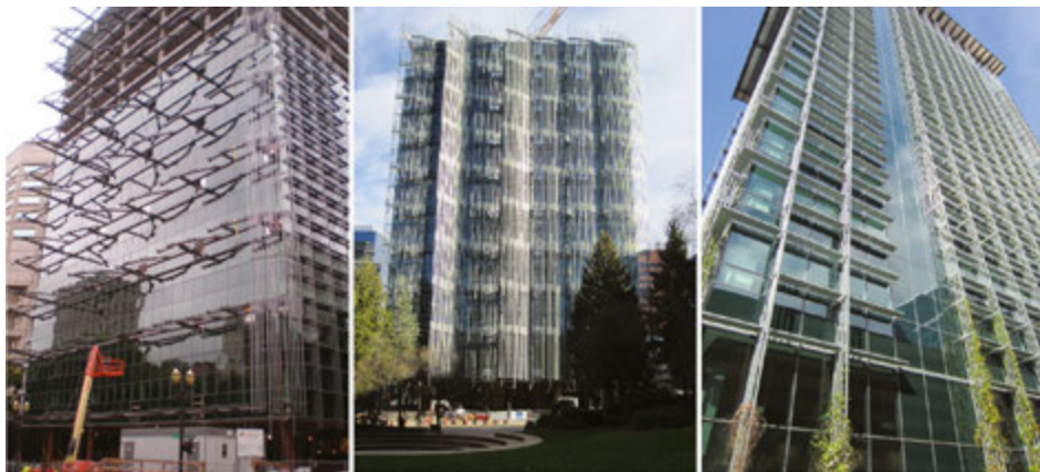
Figure 2. The Edith Green - Wendell Wyatt Federal Building during facade replacement in 2011 and after in 2012 (Middle) and 2014 (Right). Images: CC-BY-SA Another Believer.
