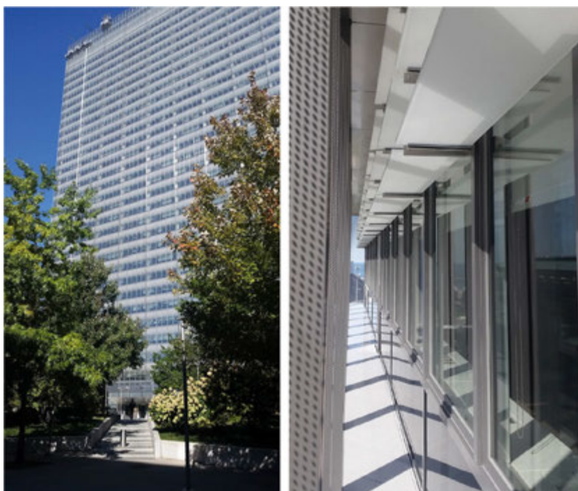
Figure 5. The Celebrezze's double-skin facades are partitioned as story-high corridors on southeast and southwest elevations. View of southwest facade (Left). View inside the corridor double-skin facade cavity (Right). Images: Author.
