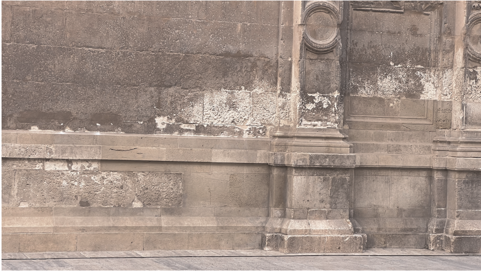
Figure 22. Limestone ashlars with varying degrees of deterioration on the facade of the bell tower of the Cathedral of Murcia (photo by the author).
