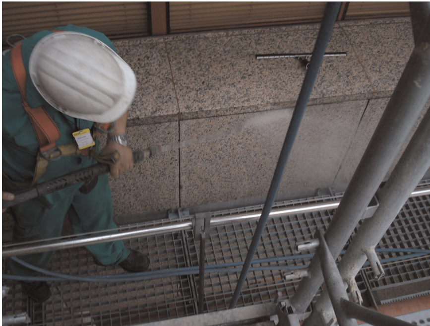
Figure 25. Cleaning operations with water jet and detergent on the pink granite cladding of a building in Madrid (photo by the author).
