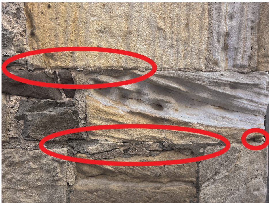
Figure 24. Detail of a sandstone wall in Soria, Spain, where cemented cuttings can be seen (photo by the author).
