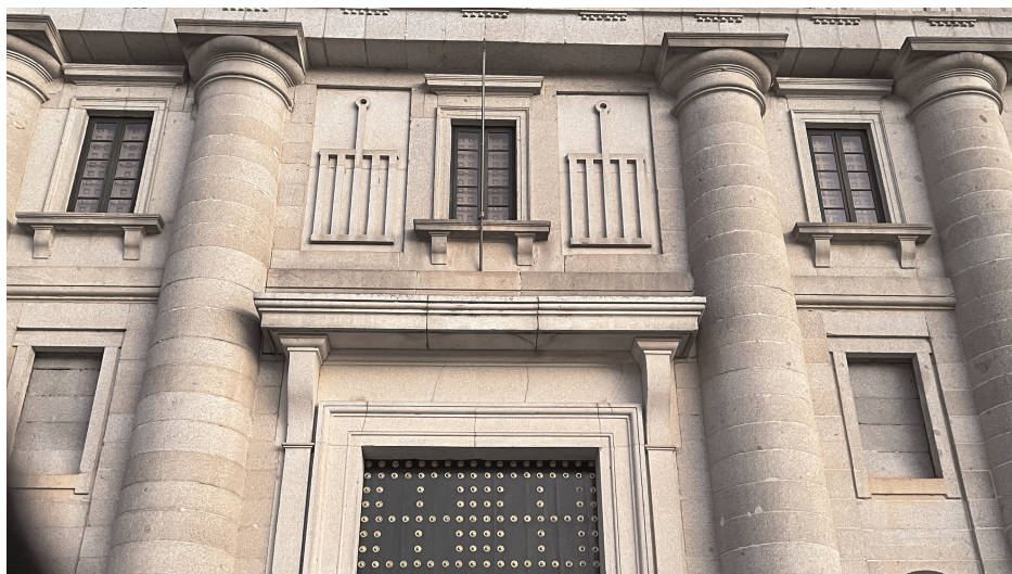
Figure 16. Fractures in the granite lintel above the main entrance to the Monastery of El Escorial, the result of a complex bending process (photo by the author [18]).
