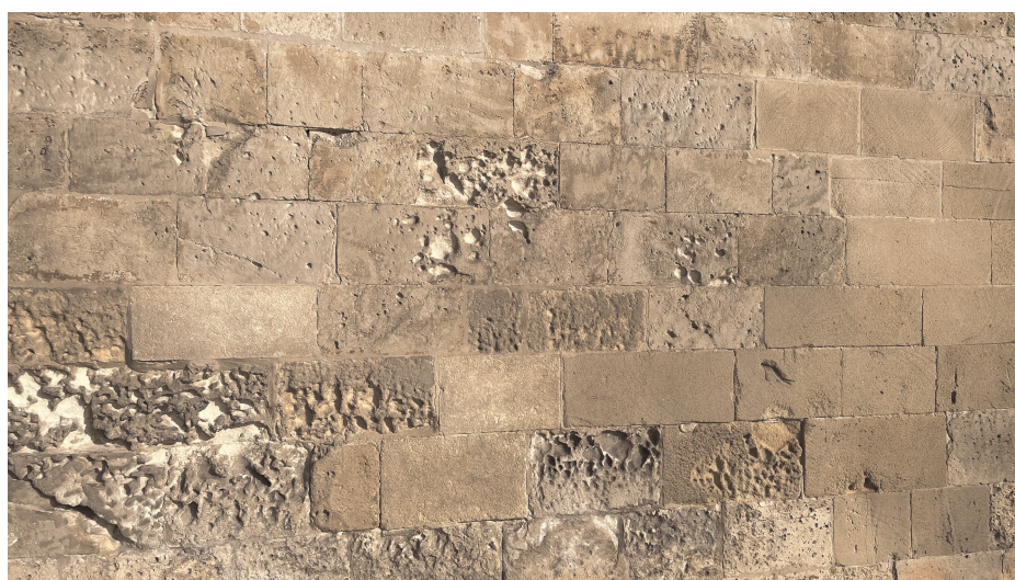
Figure 21. Sandstone ashlars from Marés on the facade of the Cathedral of Palma de Mallorca (photo by the author [29]).
