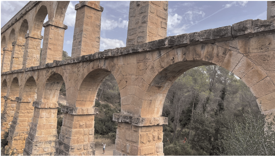
Figure 4. Roman aqueduct of Tarragona, built with limestone ashlars during the first century BC (photo by the author).
