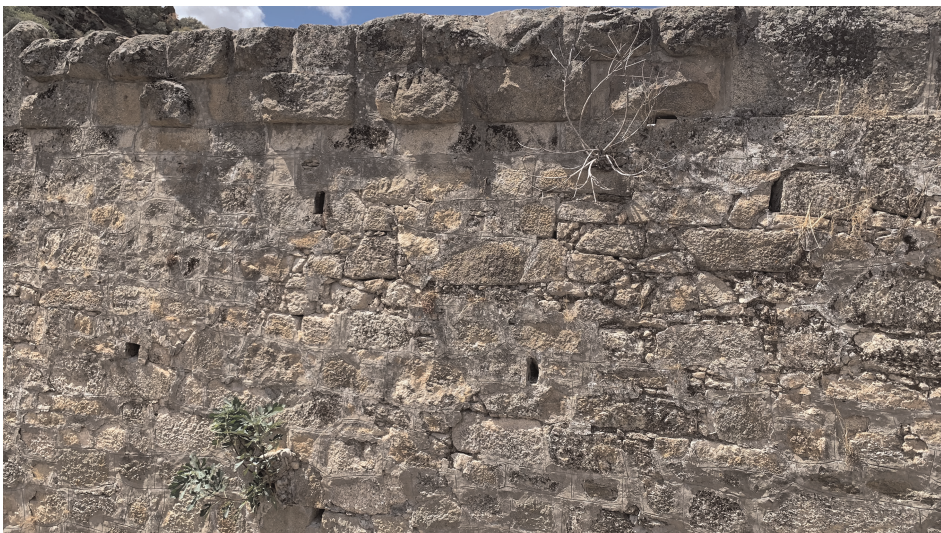
Figure 23. Granite masonry wall in Fermoselle, Zamora, Spain (photo by the author).
