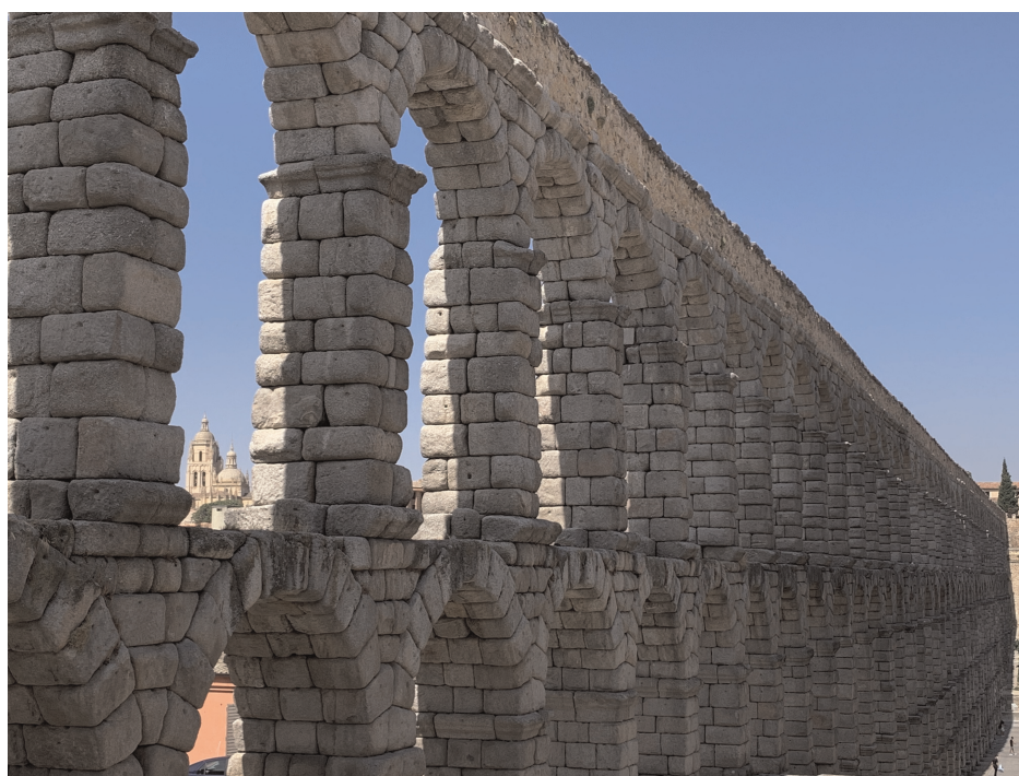
Figure 3. Roman aqueduct of Segovia, built with granite ashlars between the second half of the first century and the beginning of the second century (photo by the author).
