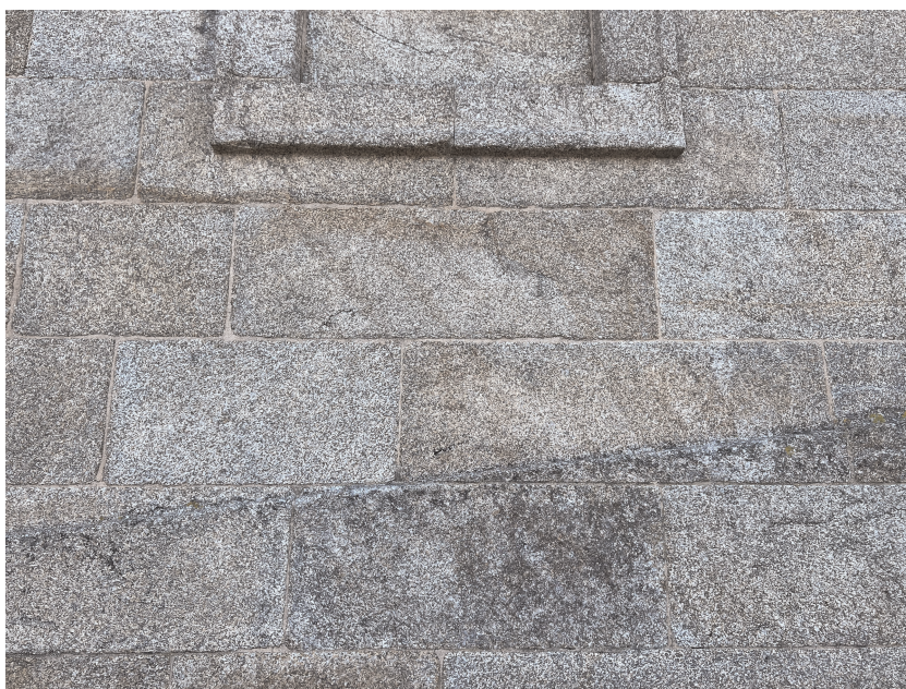
Figure 20. Granite ashlars on the facade of the Tower of Hercules (photo by the author [27]).
