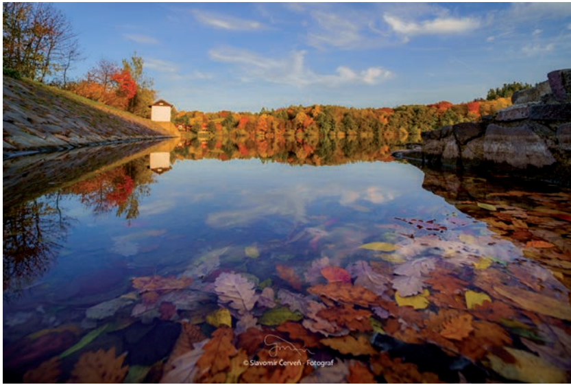
Figure 2. Great Richňava, an example of eighteenth century earth-filled structure with a height of 32 m, one of the highest of its kind in Europe (Photo: Slavomír Červený).
