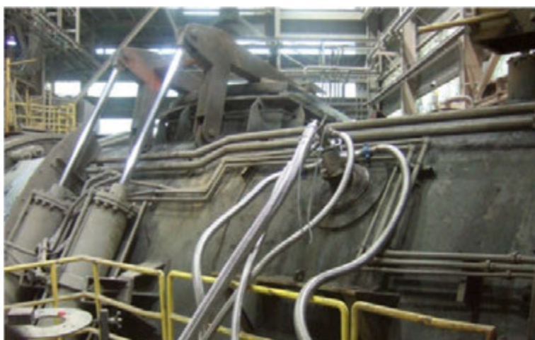
Figure 5. CoJet installed in an anode furnace [22, 23].
