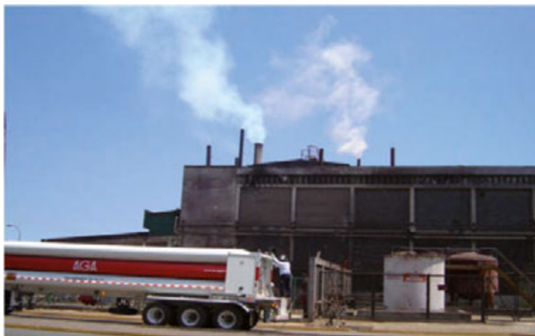
Figure 14. A hydrogen tube trailer delivering H_2 for the trials at Codelco facility [26].
