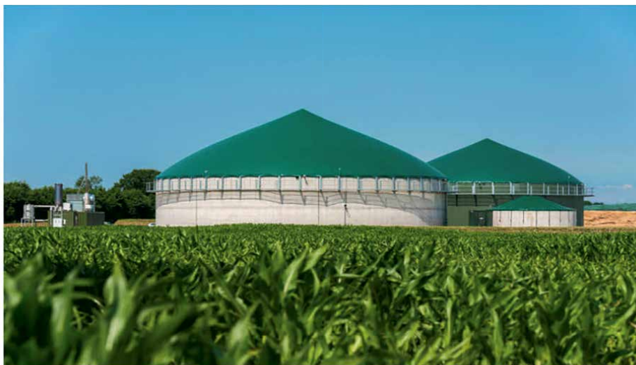
The Gorge Farm Energy Park, located in Naivasha, produces 2MW of electricity, which is more than enough to cultivate its 706 hectares of vegetables and flowers.
