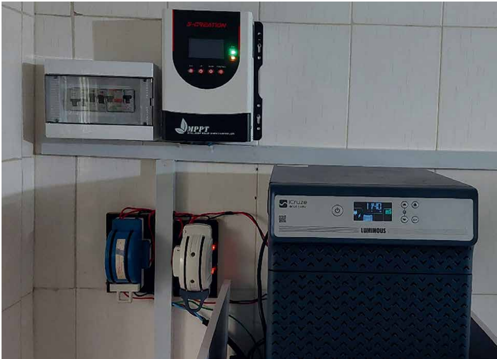
Figure 2. The solar-subpower unit anchoring the RespSS at UBTH.
