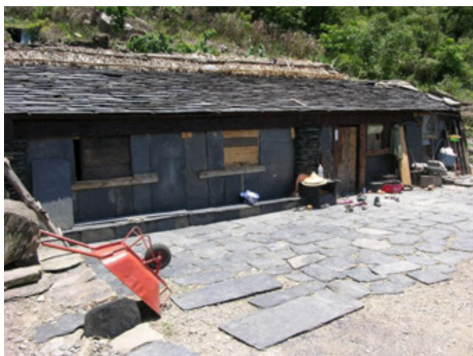
Figure 5. Taruljayaz House, Caljisi – Padain, Itapul River Basin, Taiwan [1].
