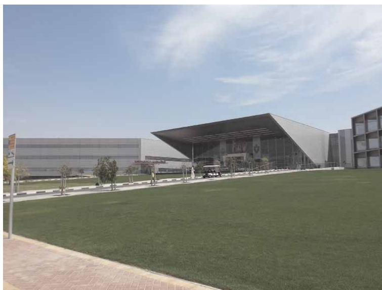
Figure 3. KHUH main buildings with the main entrance in the middle.
